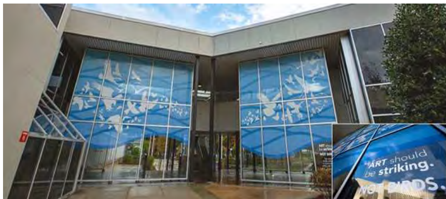
Figure 38. Perforated Vinyl on the Stockton University's K-Wing Building, Galloway, NJ
