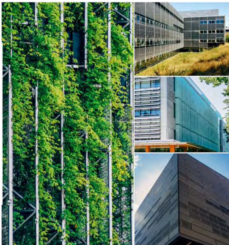
Figure 37. UBC's Bird-Safe Exteriors, Vancouver, BC Left: Mesh green wall on the Centre for Interactive Research on Sustainability. Right: Screens on the Beaty Biodiversity Research Centre (top), fins and grills on the Earth Sciences Building (middle), and zinc panels on the Campus Energy Centre.
